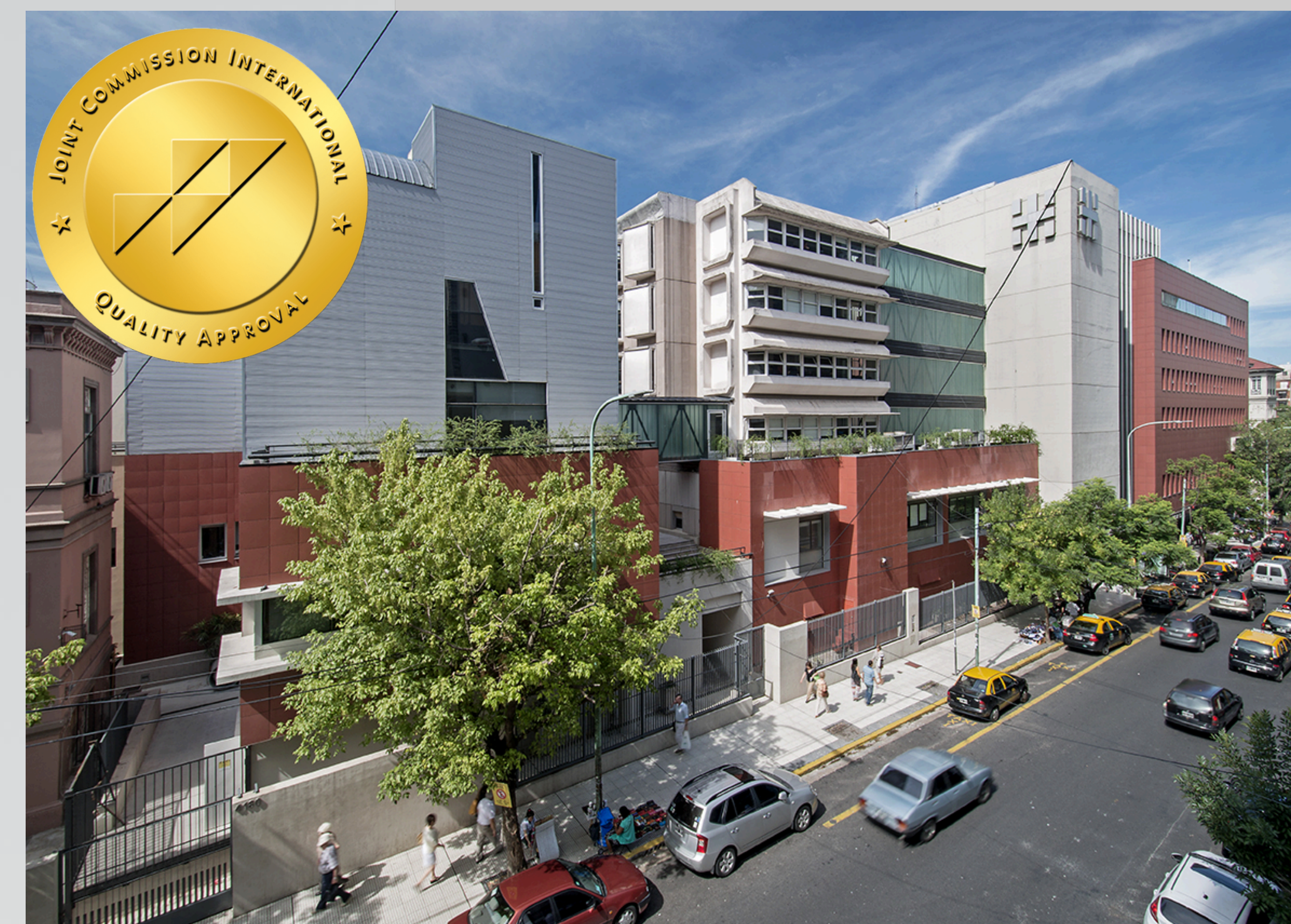
Hospital Italiano, Buenos Aires. Arg
